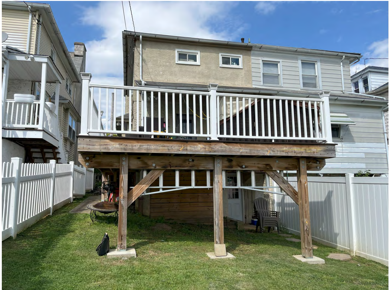
EXISTING VIEW FROM YARD
