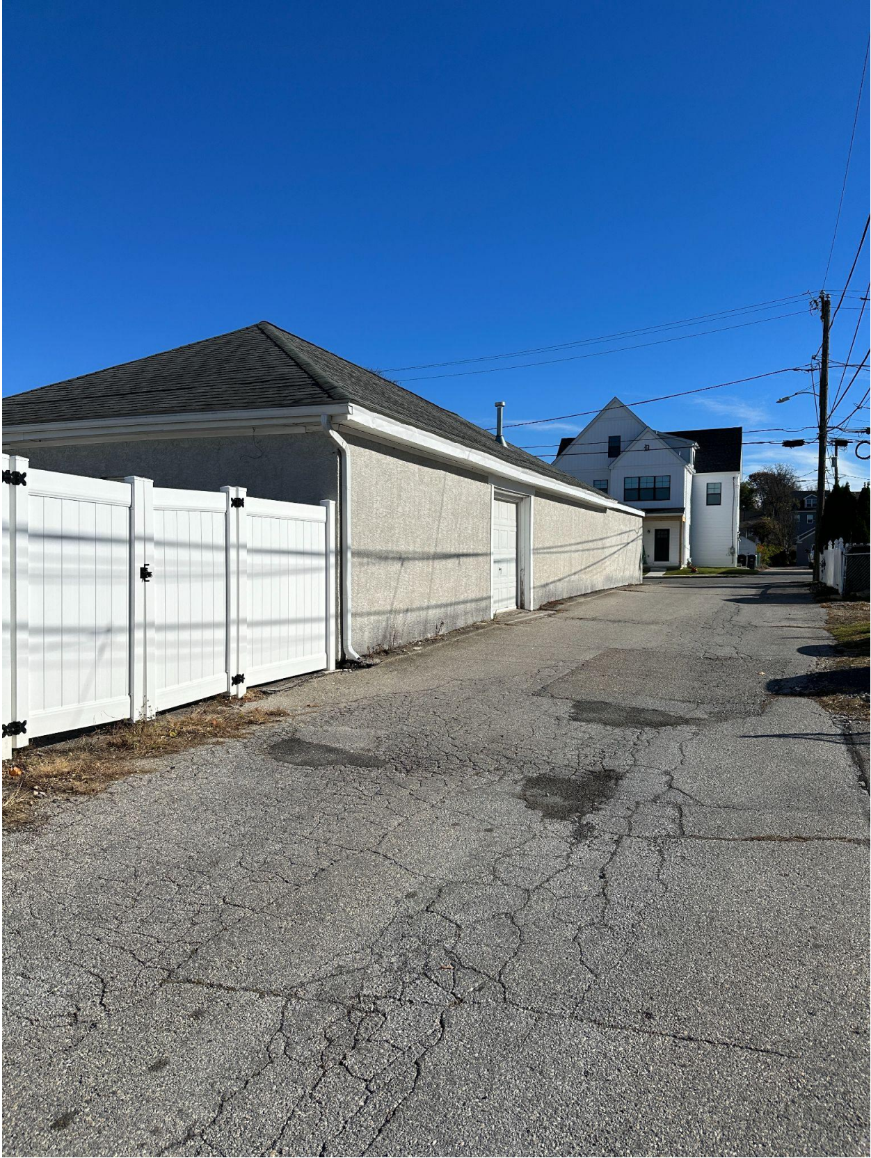
Drive Alley Behind 344 W 11th Ave - No set back
