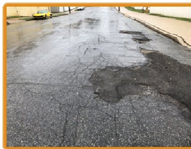
Mill & Overlay with Moderate Base Repair Jones Street (Spring Mill-E. Hector)
