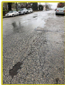
Mill & Overlay with Minor Base Repair Hallowell Street (E. 4th-E. 3rd)
