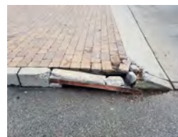
Storm Sewer Structures
