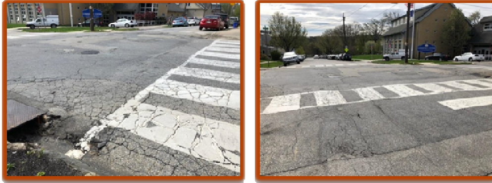
Mill & Overlay with Major Base Repair East 6 th Avenue & Harry Street
